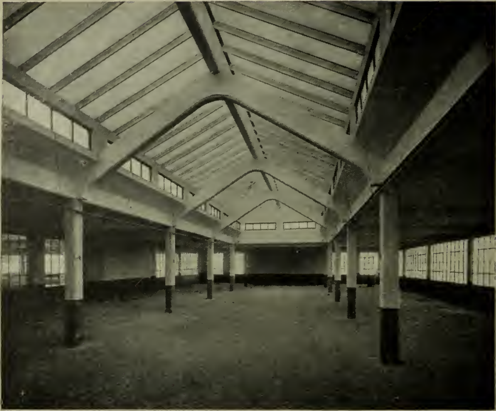
NEW WORKSHOPS FOR THE GAS LIGHT &amp; COKE CO.: MESS ROOM.
